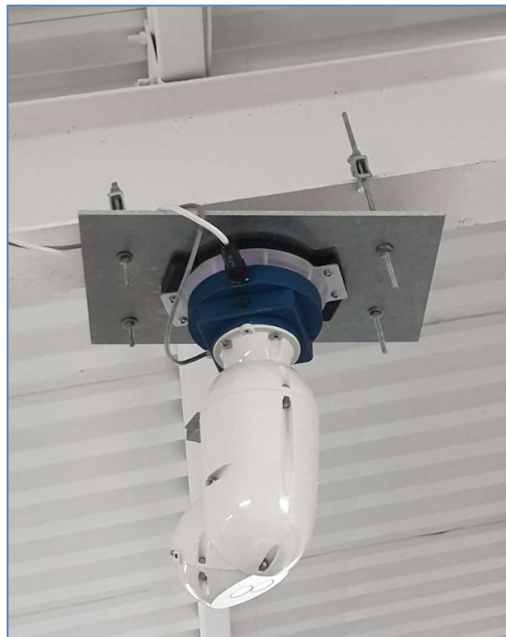
Figure 23 FiX1 installation on a customised bracket
